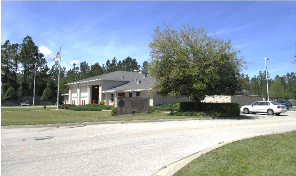
COJ fire station adjacent to proposed development.
